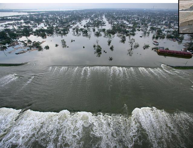
Katrina Levee Breach, New Orleans
