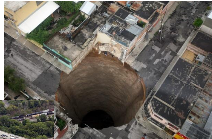
Hurricane Agatha sinkhole, Guatemala
