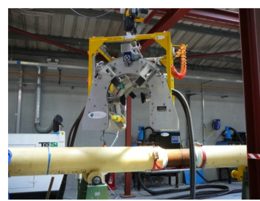
Surface cleaning Grit blasting
